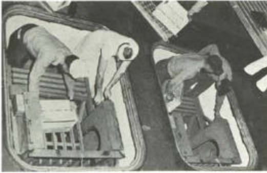
Flush deck installation
