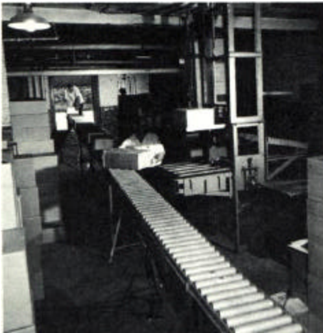
Rigid arm vertical Armorbelt® converts 5 floor old school building into an efficient warehouse.
