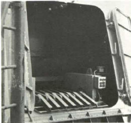
Top station 36A175 unit & deck house
