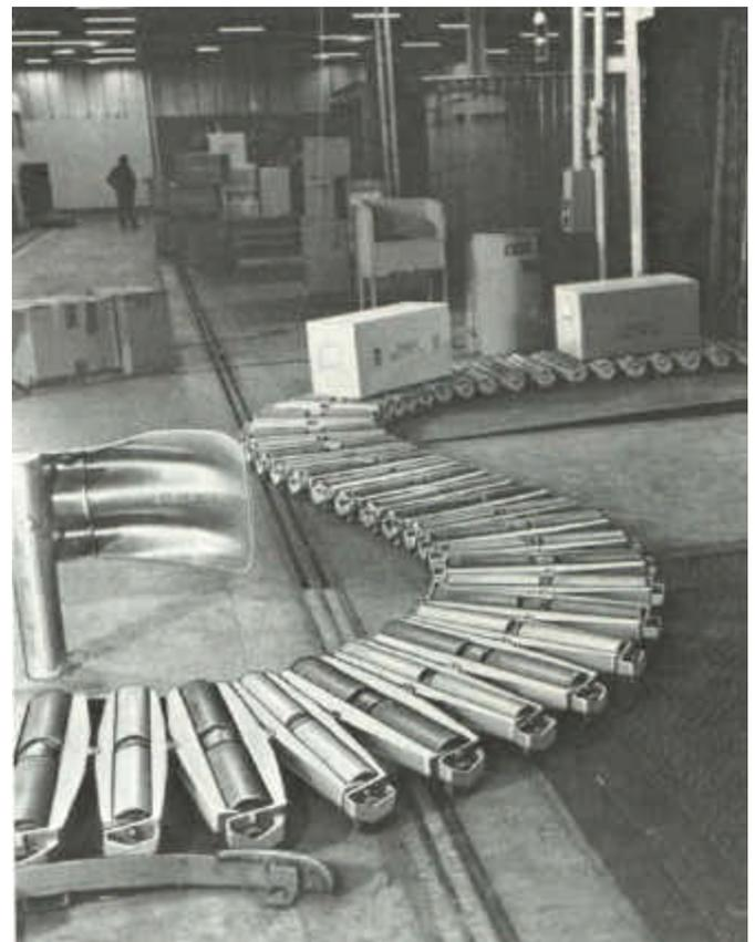
The UPC's versatile "snaking" capability enables effortless handling of luggage, packages, etc. through cramped transport routes, thus reducing loading/unloading time and employee fatigue.
