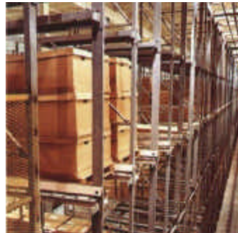
Palletflo high bay with stacker
