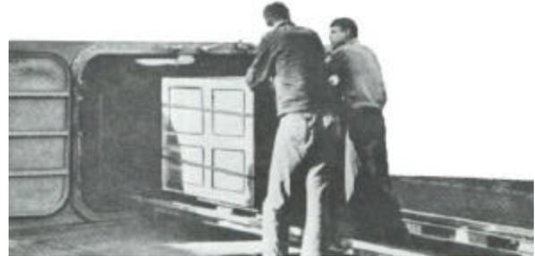
The usual Pushline, with Model RP-205 wheels, requires a push effort equal to about 3% of the load (e.g., 60 lb. Effort for a 2,000 lb. Load). Model RP-204T wheels can be used to control speed and brake the load. There usually is clear walking space between the two rails, making pallet movement safe and easy.
