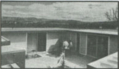
House built of 9' wide panels with pre-finished interior and exterior
