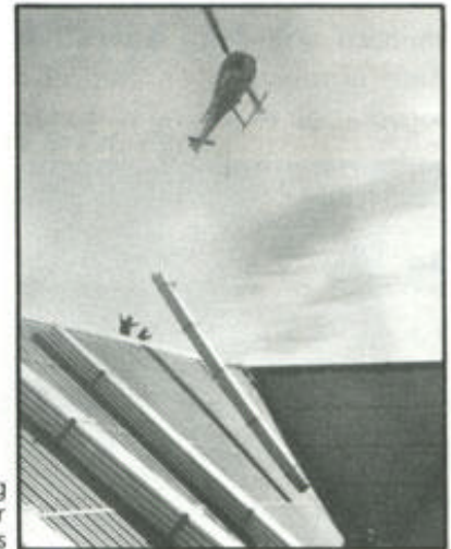
Roofing installation air cargo hangars
