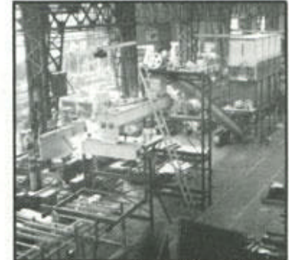
Continuous rebound line being assembled in the Kornylak plant
