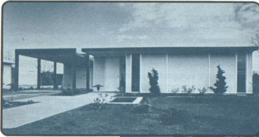
A modern insulated home assembled from 9' wide panels on edge, (Kaiser), illustrating the 1-Side-Of-A-House-In-3-Minutes* Technique.
